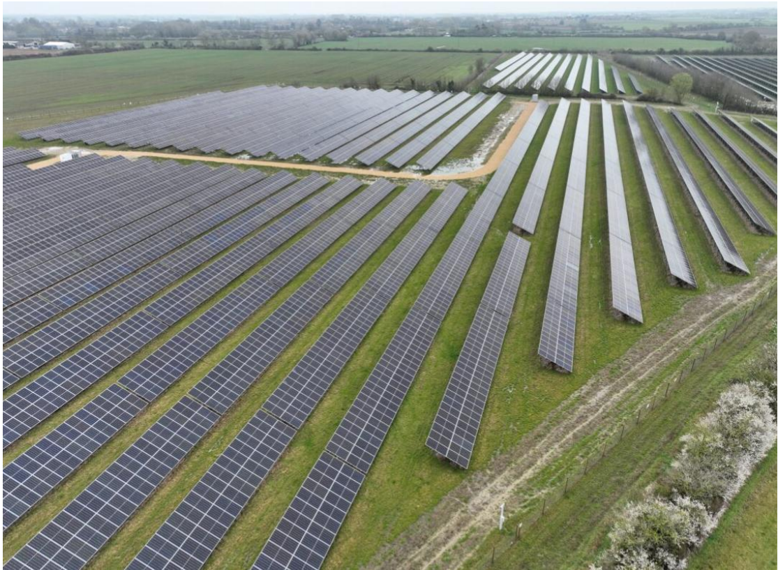
FIGURE 9.1 – EXAMPLE OF SOLAR ARRAYS
